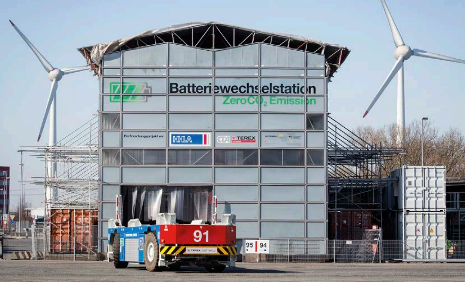
Research project BESIC at the HHLA Container Terminal Altenwerder: At the battery swapping station, the batteries of automated guided heavy goods vehicles are charged with surplus green power.
